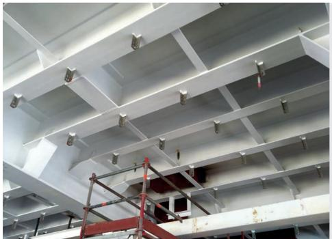
MultiGrid® is our concept of installing a grid of welded starter brackets in a set pattern over the entire equipment area as opposed to having to pre-determine, locate and provide support directly over each specific component requiring support.
